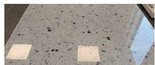
Terrazo JUNEAU Flooded
